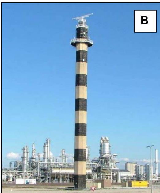
Figure 2: (a) Location of Radar Post 02 at Maasvlakte (RP2); (b) Radar Post 02; the height of the tower is 70 m.
