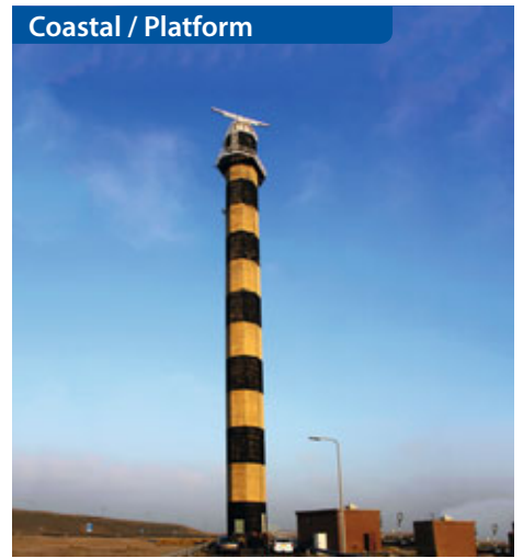
Fixed radars mounted on land can both monitor oil on surface and gather hydrographic information. A tall mounting tower is required to obtain maximum operational range.
